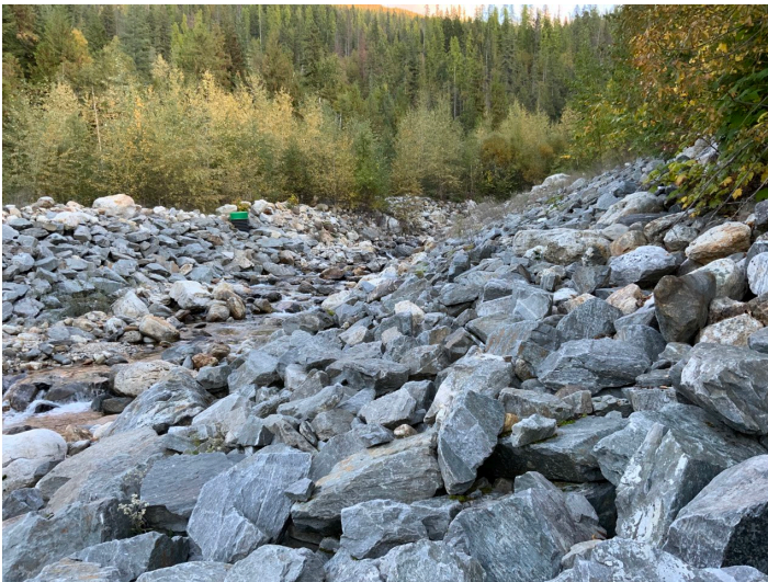
Photo 15. Looking east (upstream) at the Hummingbird Creek channel between the fan-delta apex and Highway 97A. Note the presence of large angular rip rap along the channel banks.
