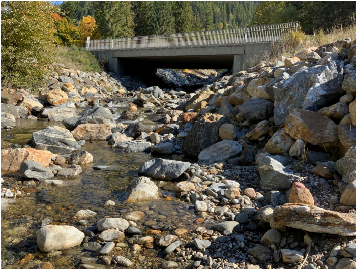
Photo 17. Looking east (upstream) at the Highway 97A bridge over Hummingbird Creek.
