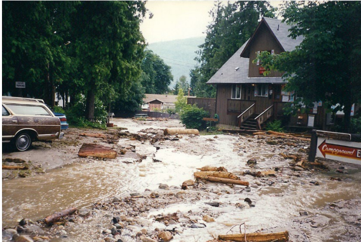
Photo 33. Looking west at 718 Swansea Point Road on the lower fan-delta and the damages from the Hummingbird Creek debris flow on July 11, 1997.
