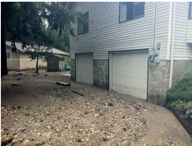
Photo 37. Looking at debris deposition at an unknown house on the lower fan-delta following the 2012 debris flood.
