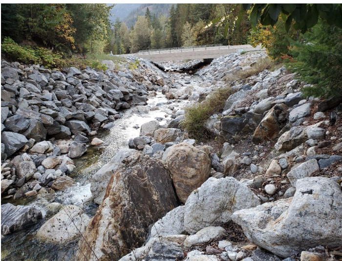
Photo 16. Looking west (downstream) at the Highway 97A bridge over Hummingbird Creek.
