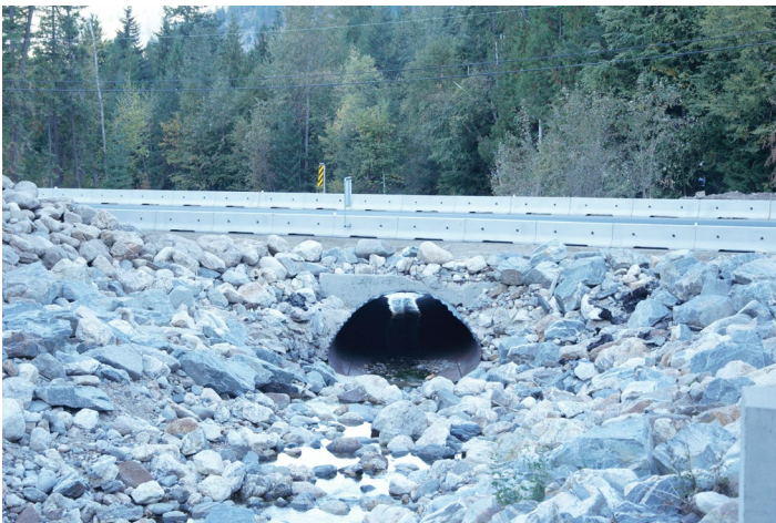
Photo 18. Looking west (downstream) at the former culvert under Highway 97A bridge at Hummingbird Creek. Note the difference at the Highway 97A crossing compared to Photo 16.
